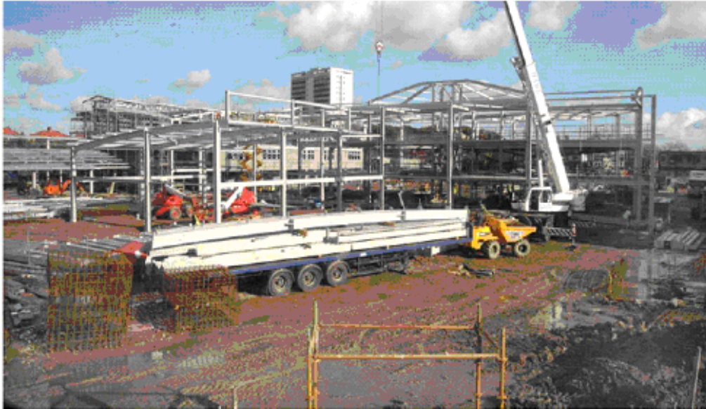
Construction of school
